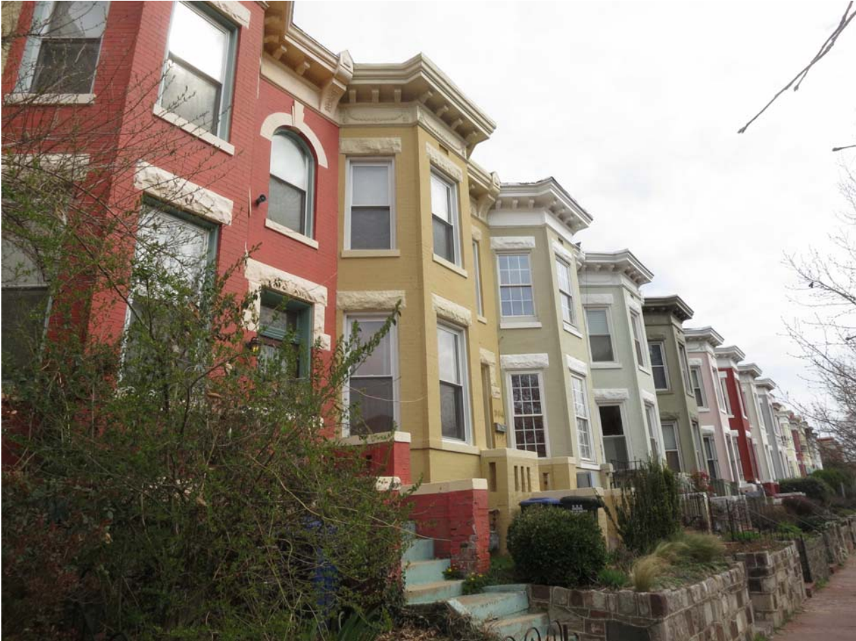
Figure 2. Classical Revival rowhouses on the 300 block of G Street, NE, north side, looking east.
