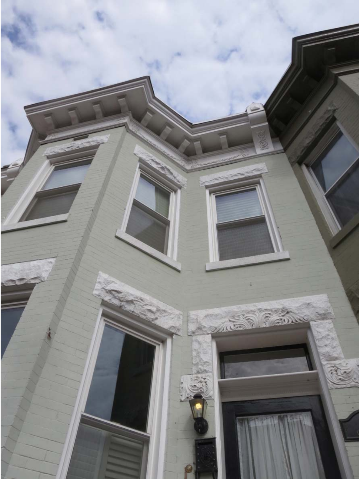
Figure 4. Cornice detail, Classical Revival rowhouse, 308 G Street, NE
