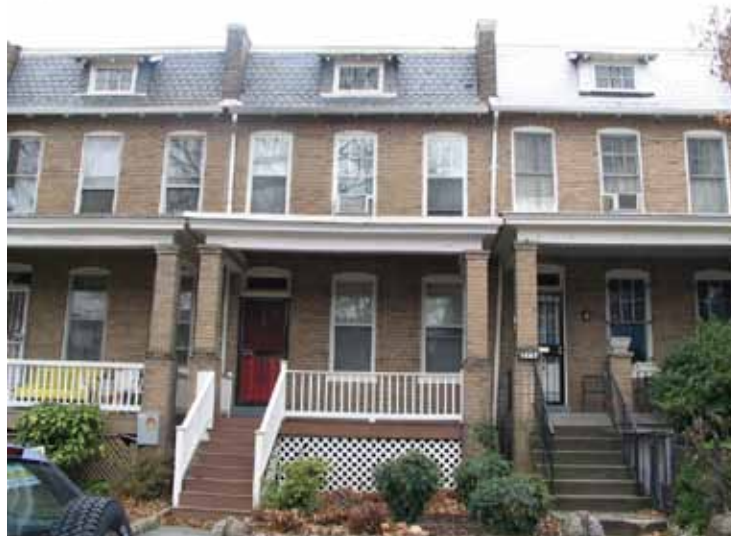
1609 E Street, SE: Jameson (1919). Brick porch-front house with mansard roof, fish-scale slate tiles, shed dormer with overhanging eaves and exposed rafter ends.
