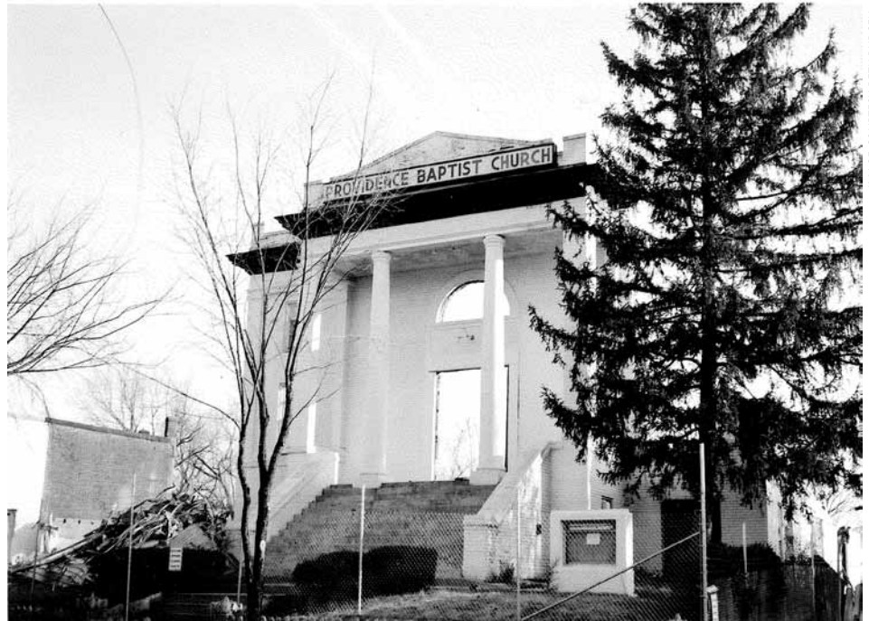
Providence Baptist Church during demolition in 2005.
