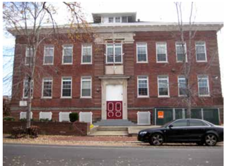
Developer CAS Riegler proposes to convert the 1903 Edmonds School at 901 D Street, NE to condominiums and four townhouses.
