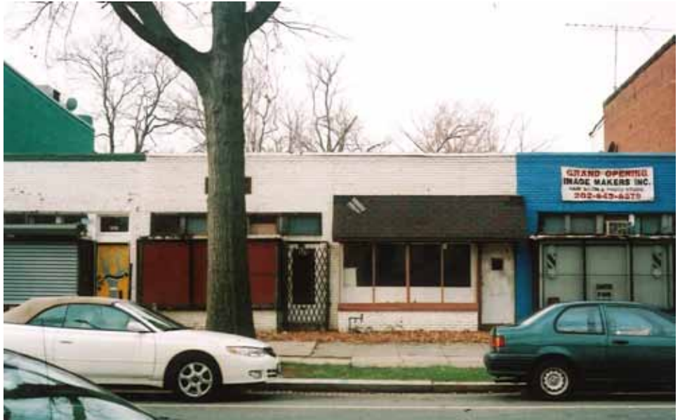
Photograph of 243–249 15th Street, SE (demolished); 243 appears on the right.
