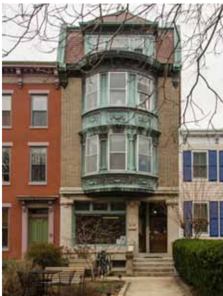
The William Penn House at 515 East Capitol Street is an unusual stop on this year's House and Garden Tour.
