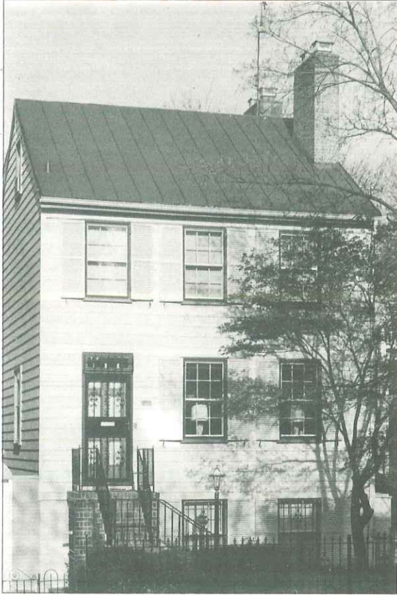
This 1821 frame house, with its unadorned flat front, gabled roof, and six-over-six windows, is a rare example of the Federal style on Capitol Hill. Unlike Georgetown, most of Capitol Hill developed after the Civil War by which time taste had turned to more decorative expressions.
