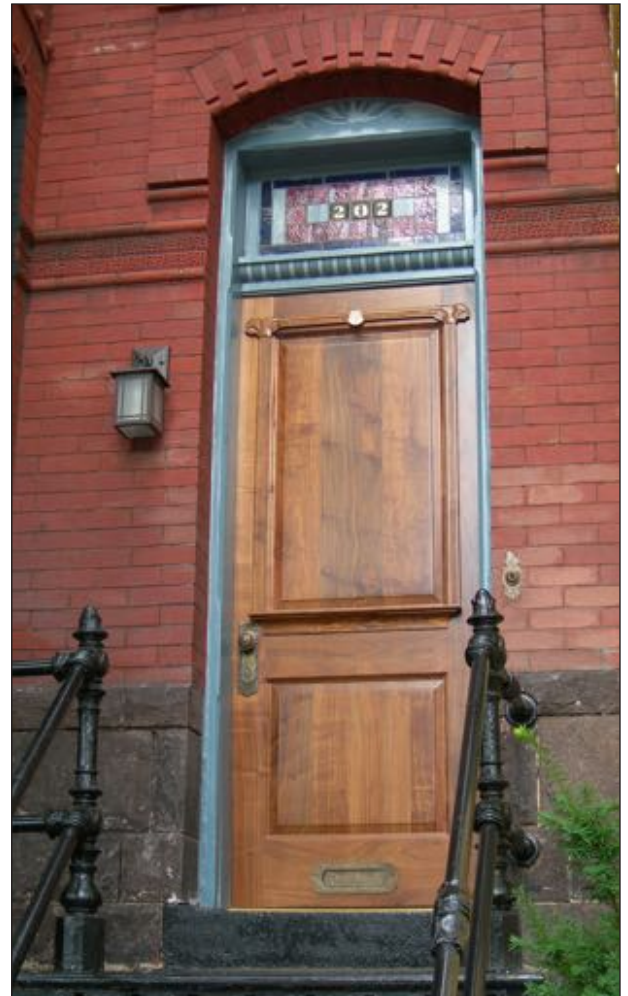
This replacement door replicates the material and detailing of the original door.
