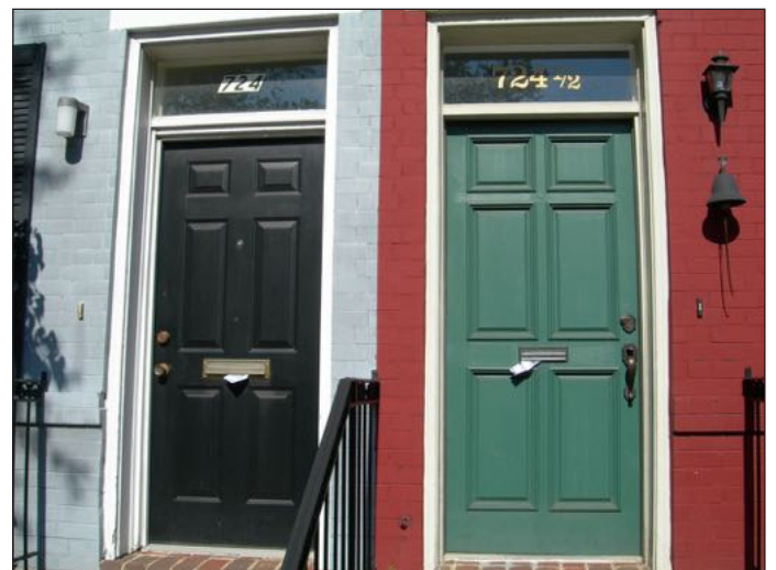
The fiberglass door on the left has flattened panels and no molding. The wood door on the right, with deeper panels and raised moldings, is a better match for the replacement of an historic door.
