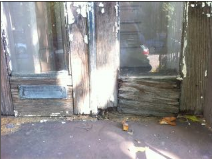
The bottom rail and side stiles of these doors are severely deteriorated, requiring reconstruction with new wood elements or wholesale replacement.
