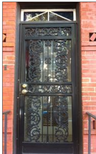
The security gate on the left obscures the building's door. The security bars on the right are integrated into the wood doors, rather than covering them.
