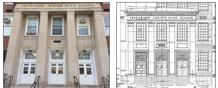
The replacement doors on this historic school building were based on the design shown in the original construction drawings.
