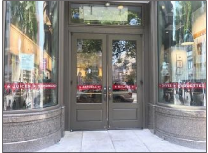
The lower panels of these doors align with the height of the storefront base to present a unified appearance.
