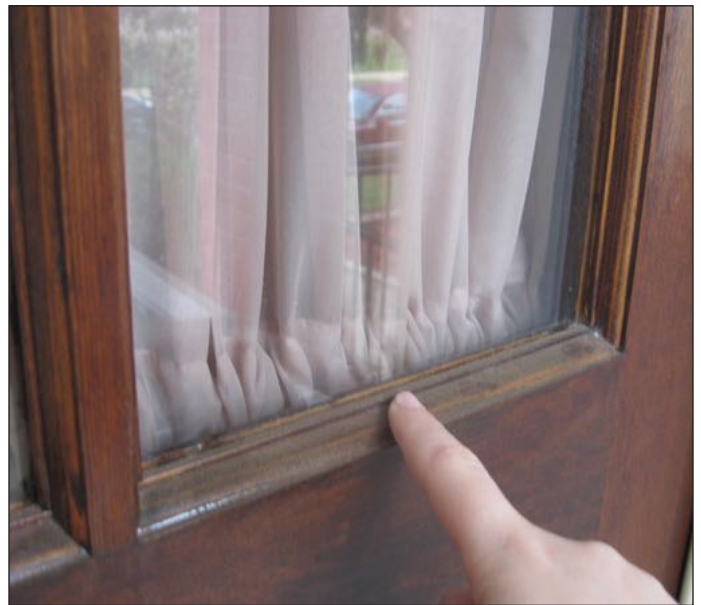
This door has wood molding around each pane that can be removed for the insertion of replacement glass.
