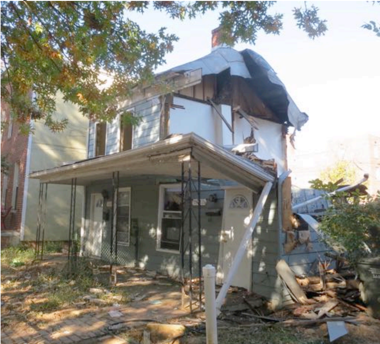
During demolition in 2016:
