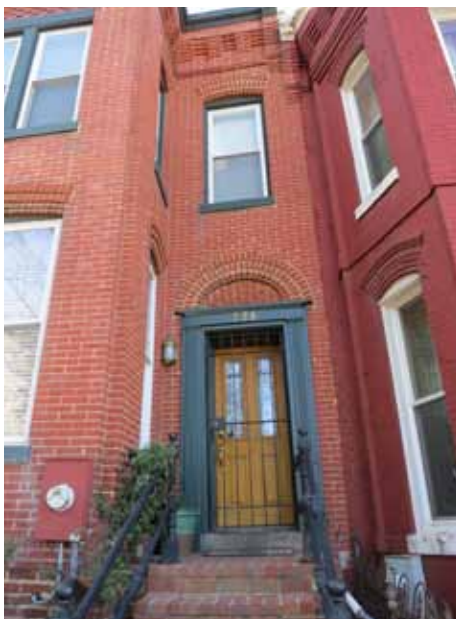
Groff building at 528 4th Street, NE.
