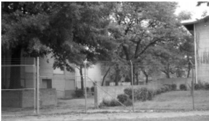
Kentucky Courts: September 2001. View from Kentucky Avenue.
