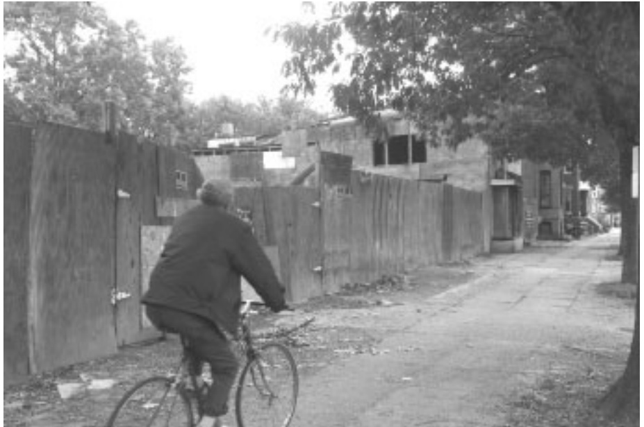
Instead of stabilized historic structures, a gaping hole stands in the 1200 block of Pennsylvania Avenue SE. The frame buildings at 1224 and 1226 Pennsylvania Avenue (in the background) will be the next to be demolished by the same owner's intentional neglect.
