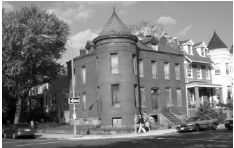
Your assistance is needed in identifying vacant properties. Boarded up and unoccupied structures, such as these houses, are examples of nuisance properties. Top, 221-223 11th Street, SE. Bottom, 1000 C Street NE
