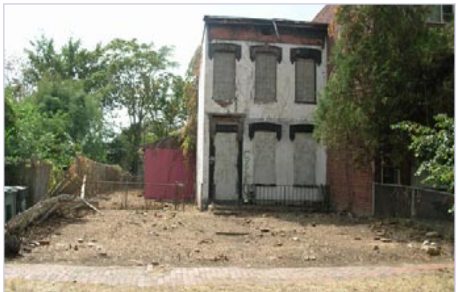
1525 E Street, SE, before (left) and after (above). Photos: Gary Peterson
