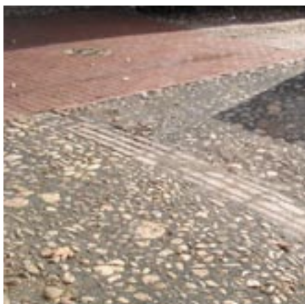
Above: Before (top) and after photos of the alley. The original cobbles were saved and relaid.
