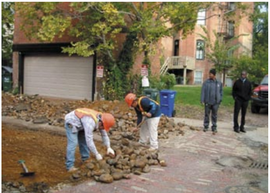
Right: The deteriorated surface of the historic alley in the 300 block of A Street SE is removed by a Capitol Paving Co. crew.
