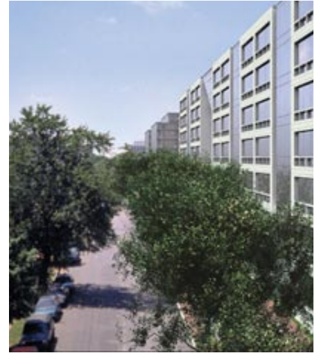
Station Place on 2nd Street NE is across the street from modest rowhouses, without adequate buffering.
