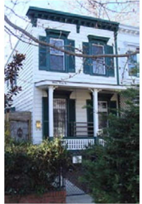
1121 G Street, NE, and its neighbor were constructed in the mid-nineteenth century with five entrances and extensive backyards
