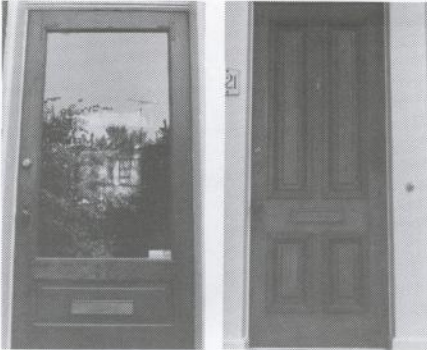
Top left The two-common Colonial-type door knocker (on a six-panel cross-and-bible door, naturally) contrasted with a door and knocker, right, at 121 Fifth Street, S.E. more appropriate to Victorian-era buildings. This photo at 121 Fifth Street also illustrates a bolection molding clearly.
