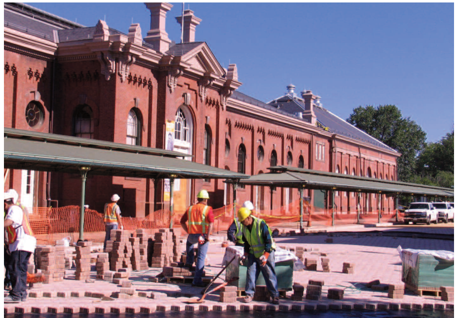
Finishing the cobblestones
