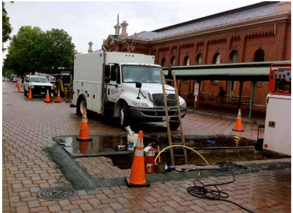
Gas line repairs at Eastern Market.
