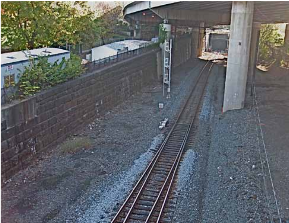
Current CSX tunnel at New Jersey Avenue where two tracks merge to one.
