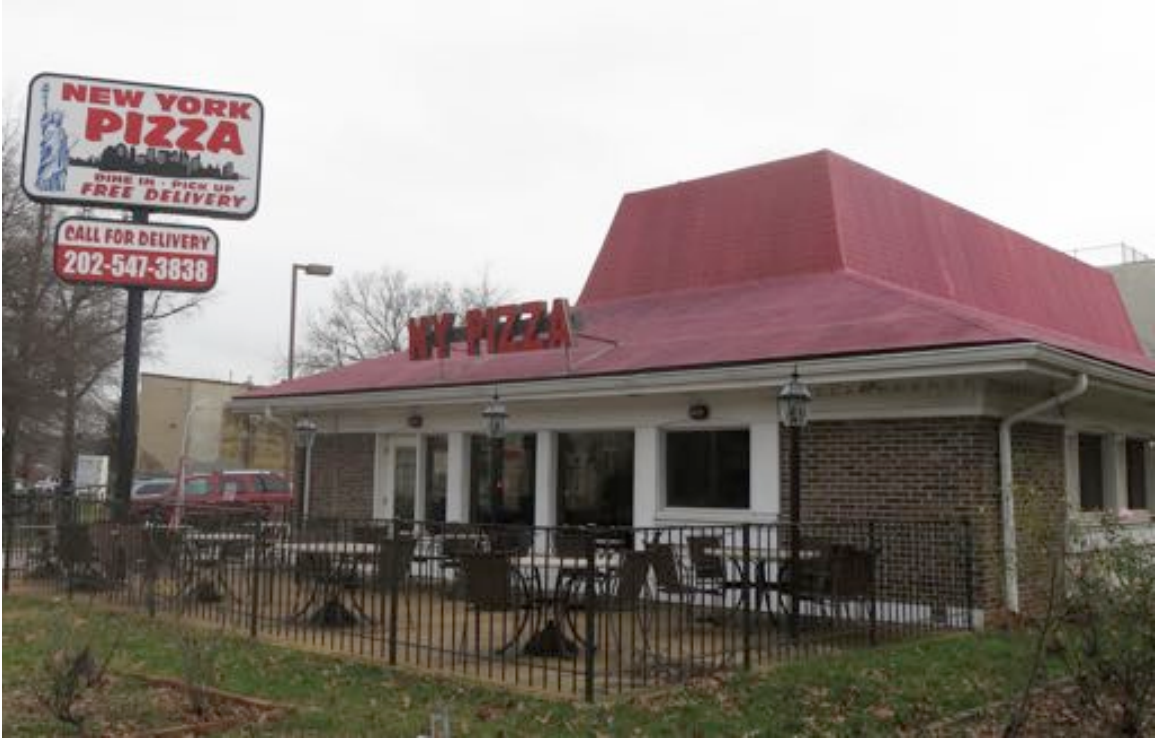
New York Pizza, 1401 Pennsylvania Avenue, SE, north elevation with pylon sign, looking southeast
