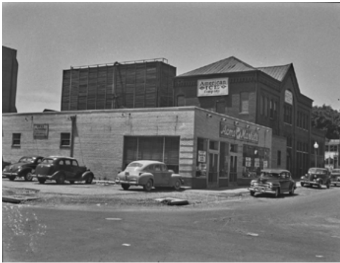
LEFT: 1515 F Street in 1949 as the American Ice Co. building; RIGHT: The site today houses Azeeze Bates Court.
