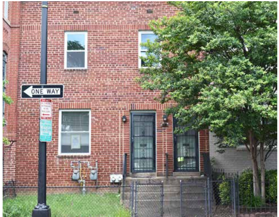
The building at 810 C Street NE will be demolished and replaced.
