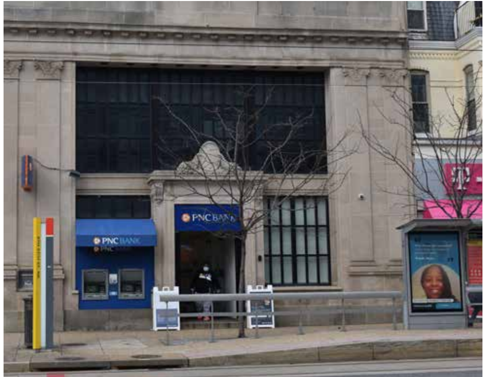
The PNC Bank building at 800 H Street NE was designed by B. Stanley Simmons.
