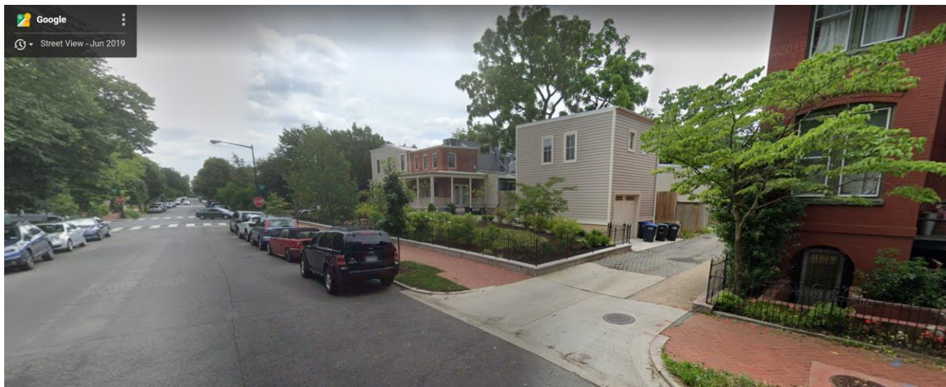
Figure 1. 401 11 th St SE garage (HPA 15-498) Looking east down D St SE to 11 th St SE. Google Maps screenshot from June 2019.
