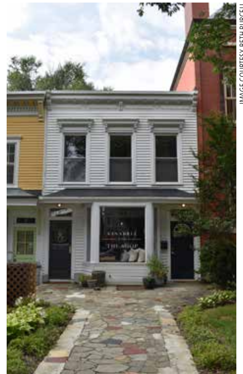
A three-story addition is proposed at the rear of 409 East Capitol Street SE.
