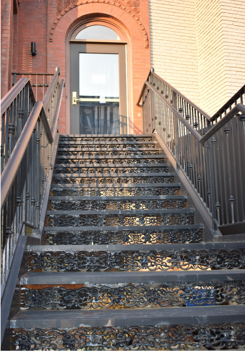
Figure 1. Detail of one of the second story entrances, 227 Massachusetts Avenue, NE
