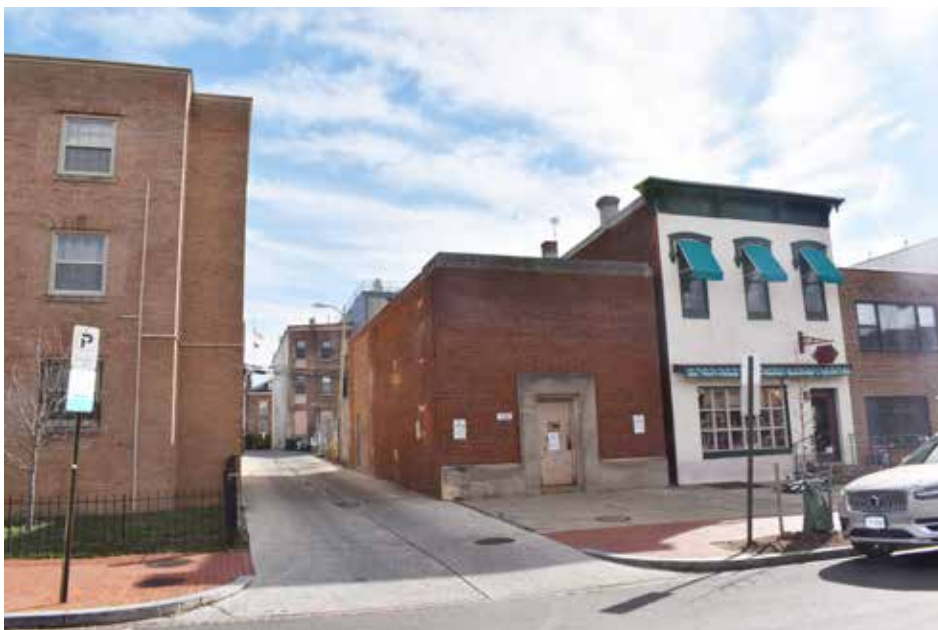
The former Pepco substation at 732 7th Street SE.
