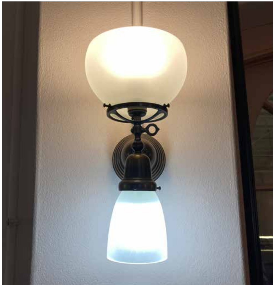
Combination gas and electric fixture in the Eastern Market manager's office.
